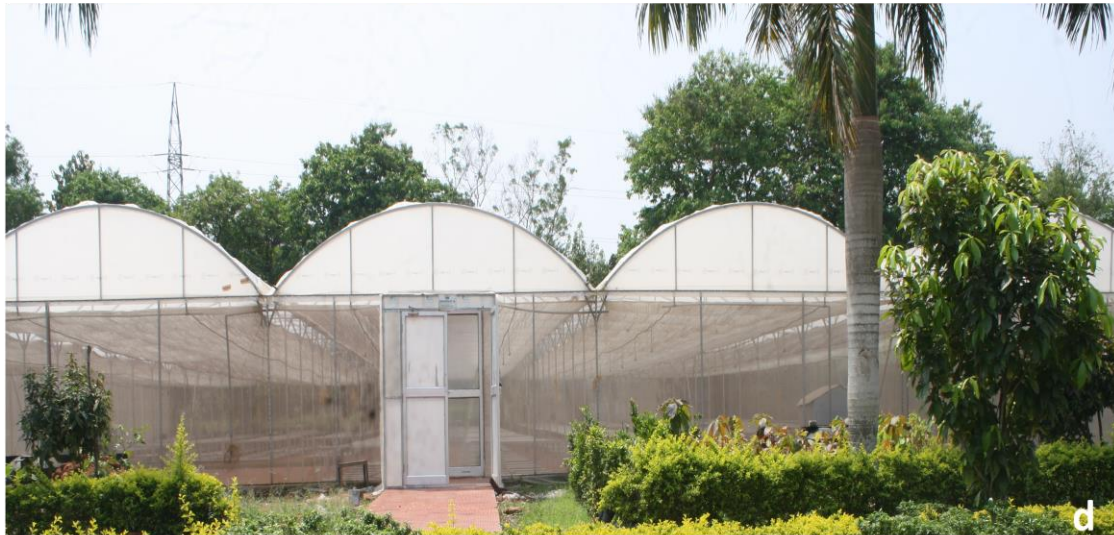
Fig. 1 Different sections of the banana plantlet production facility.
